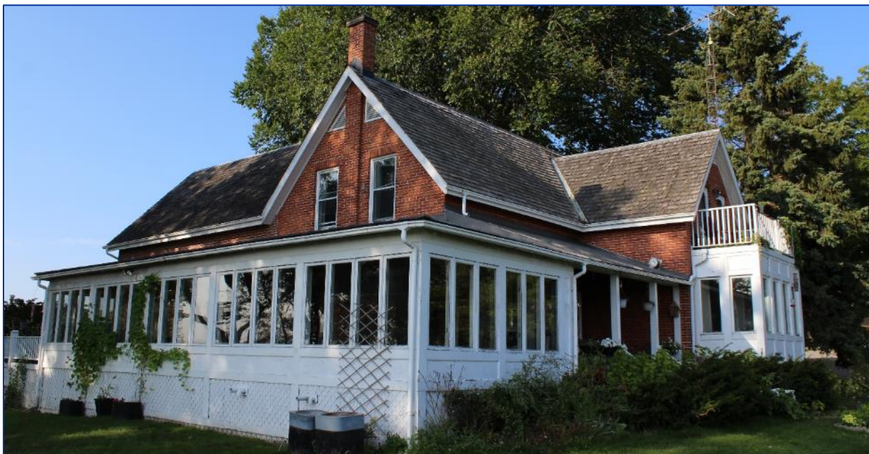
Figure 54: View north at the back of the Farm House.
