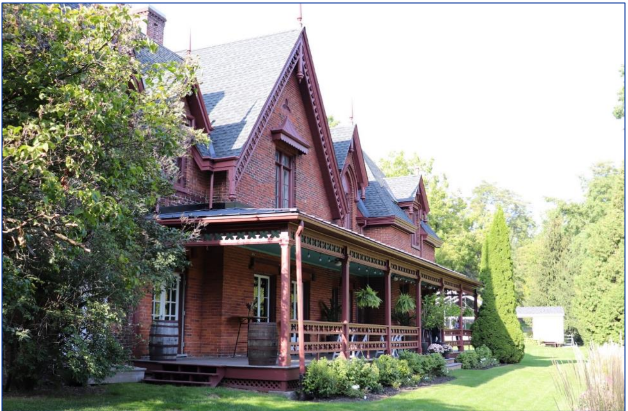
Figure 49: View northeast at the veranda on the back of the Big House.
