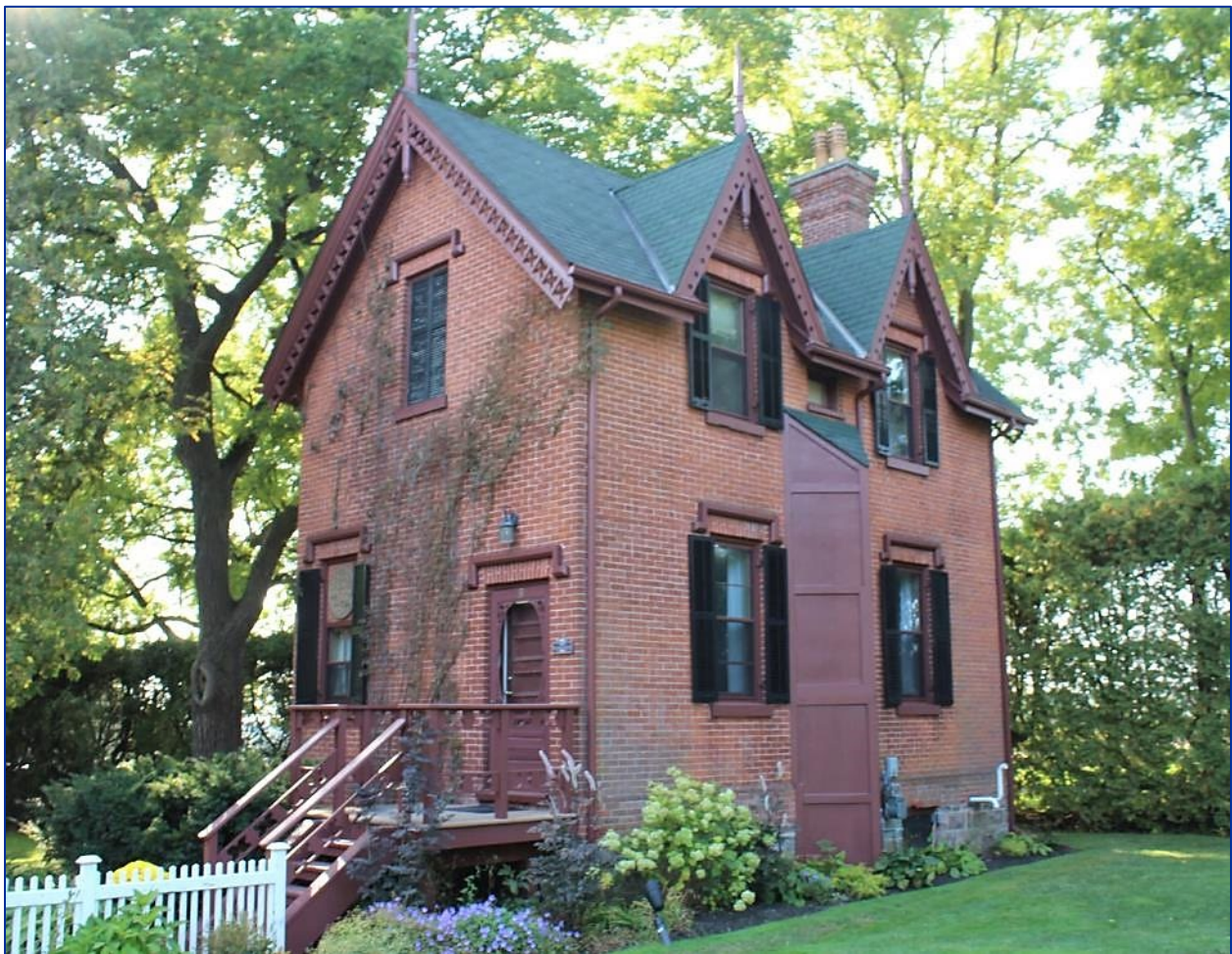
Figure 50: View west at the front and side of the Billiard House.
