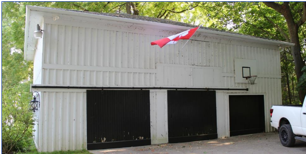
Figure 74: View south at the stable.
