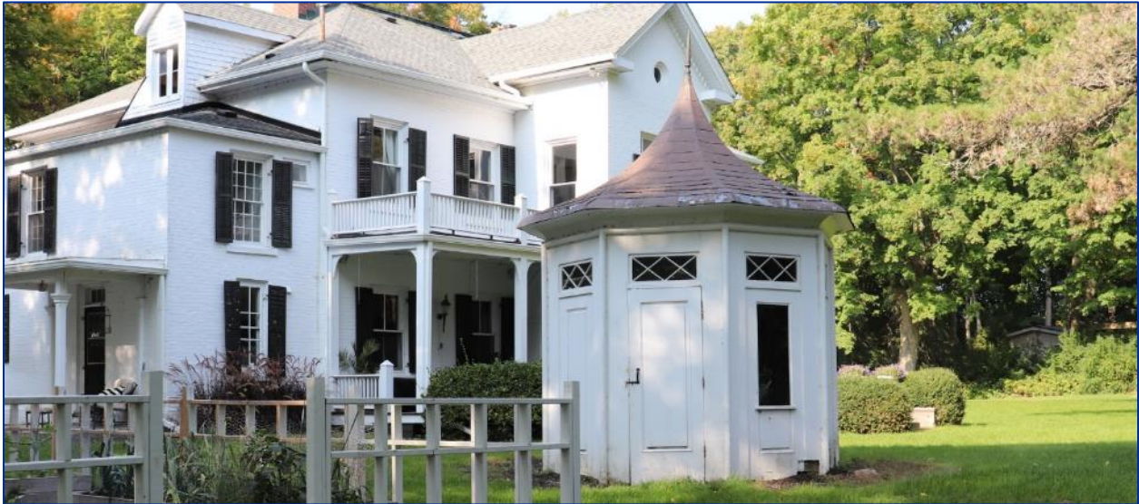
Figure 76: View northeast at Gazebo 1.
