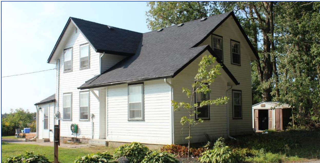
Figure 55: View west at the Lilac Lodge.
