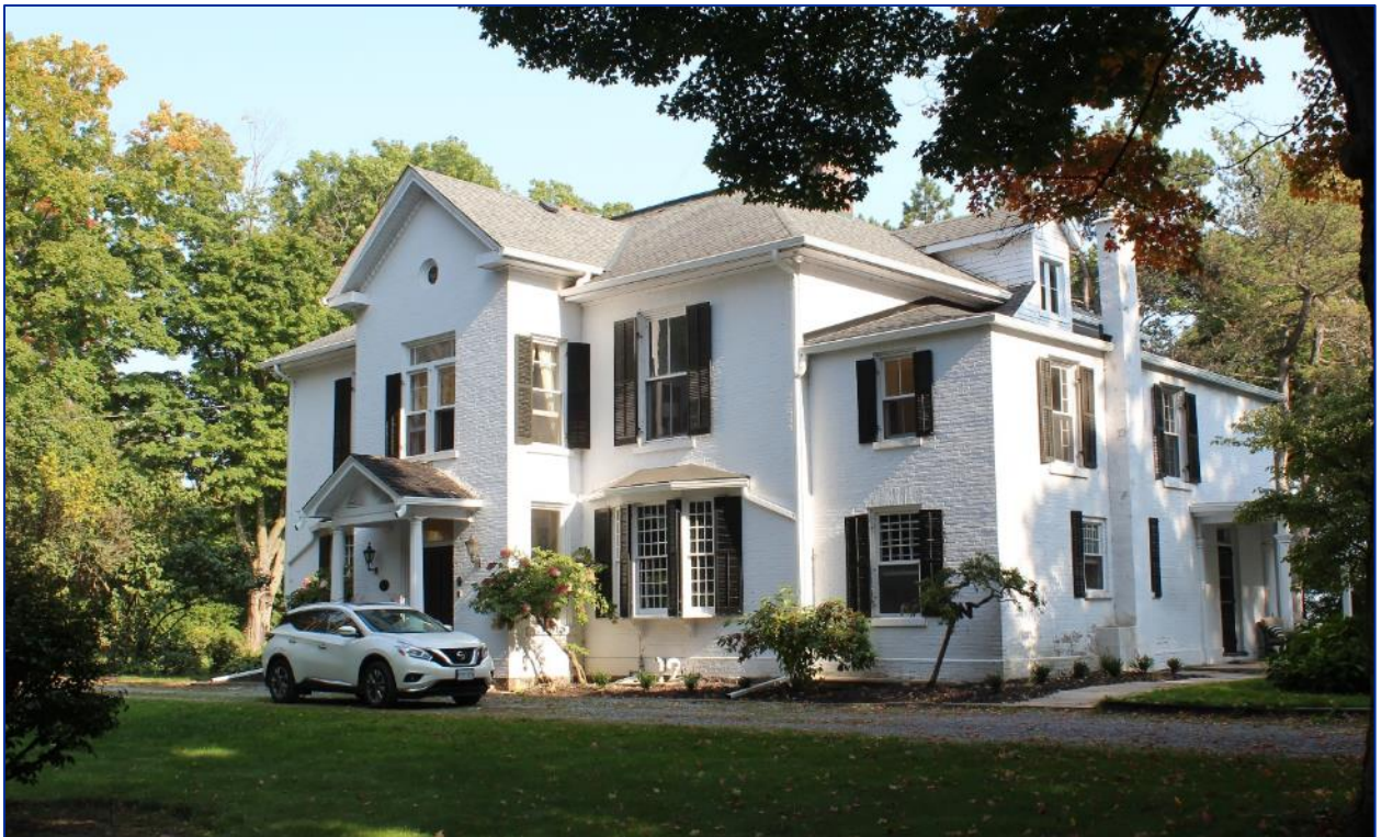
Figure 73: View east at the front and west side of Penryn Homestead.
