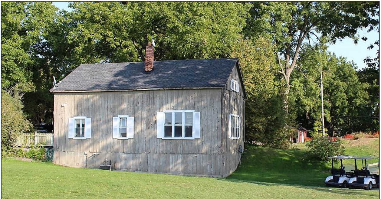
Figure 61: View east at the Golf Course Building.
