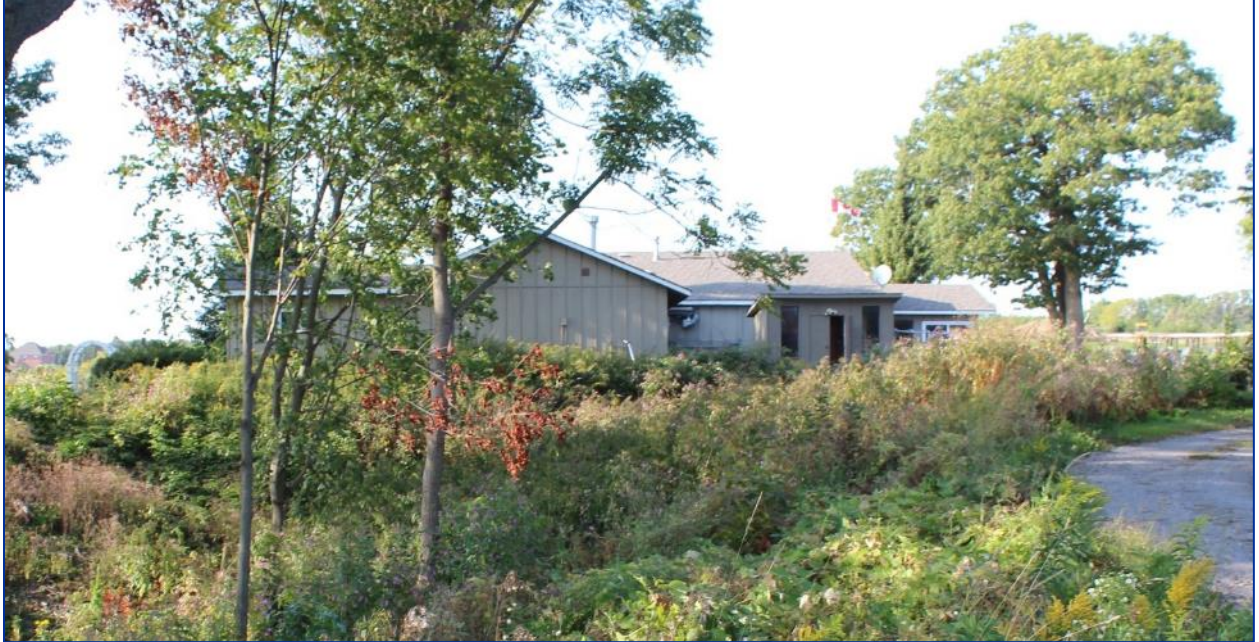
Figure 60: View north at the back of the Golf Course Clubhouse.
