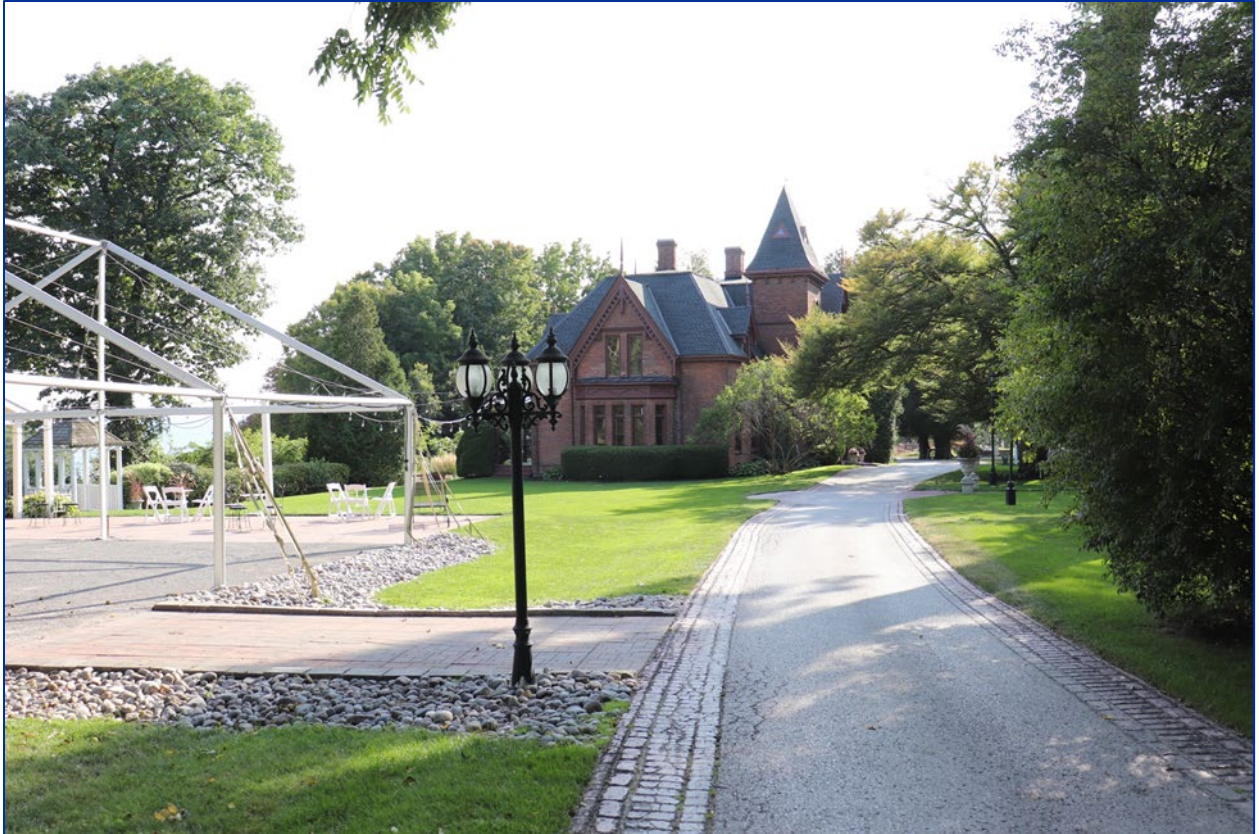
Figure 33: View southwest of the seasonal wedding pavilion and Big House.
