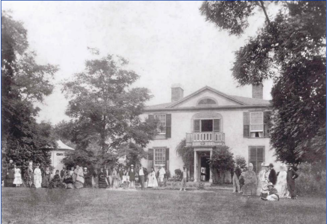
Figure 10: South elevation of Penryn Homestead c. 1890 before renovations (Archives of Ontario, cropped).
