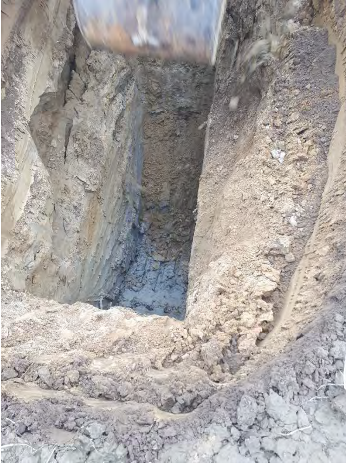
Photo of Subgrade Soils
