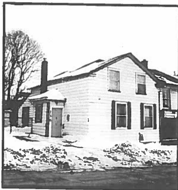
Peter John Stokes Consulting Restoration Architect
