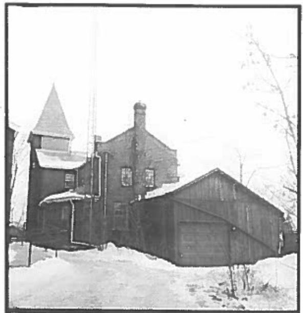
Peter John Stokes Consulting Restoration Architect
