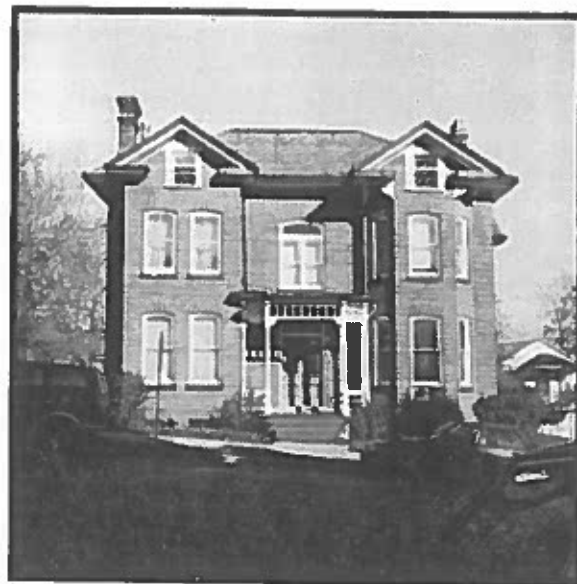
Peter John Stokes Consulting Restoration Architect
