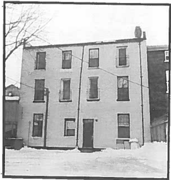
Peter John Stokes Consulting Restoration Architect
