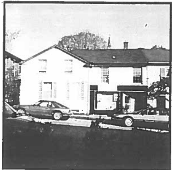
Peter John Stokes Consulting Restoration Architect
