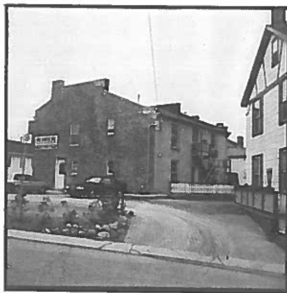
Peter John Stokes Consulting Restoration Architect
