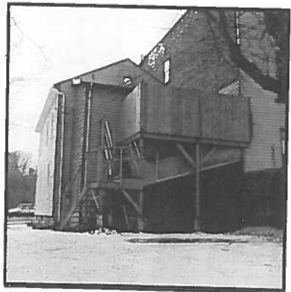
Peter John Stokes Consulting Restoration Architect
