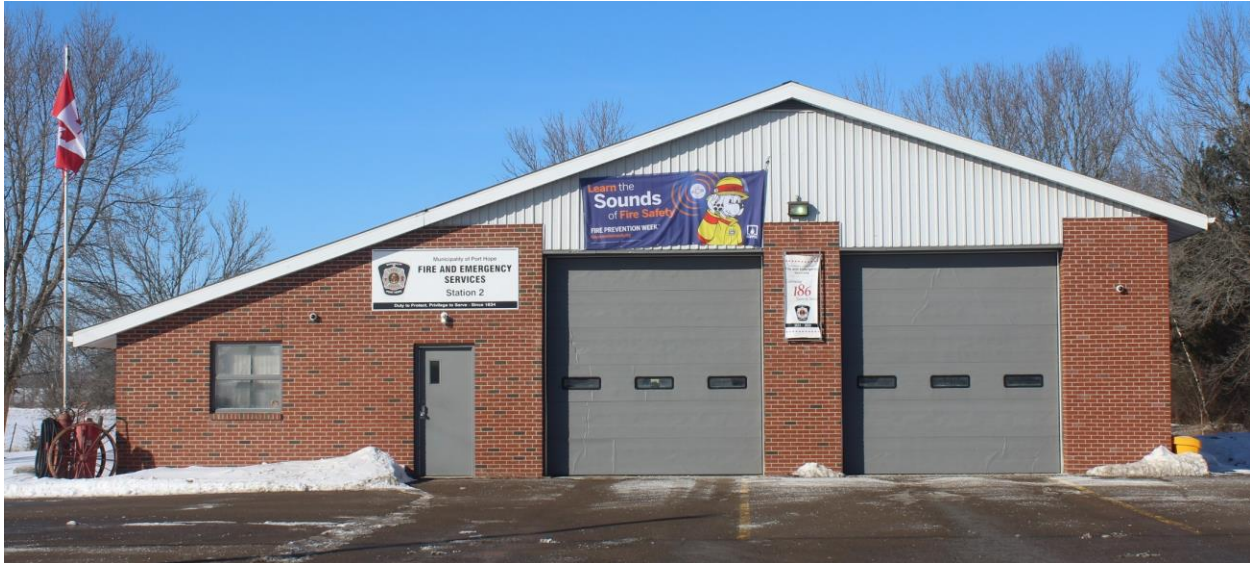
Figure 22: Fire Station 2 (Welcome)
