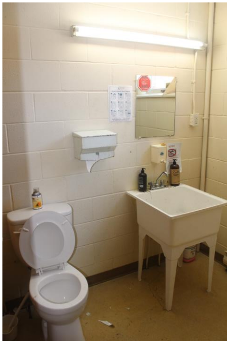
Figure 24: Picture of washroom at Fire Station 2.
