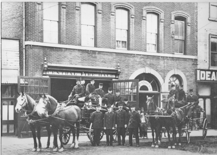
Figure 2: Exterior of the Central Fire Station.
