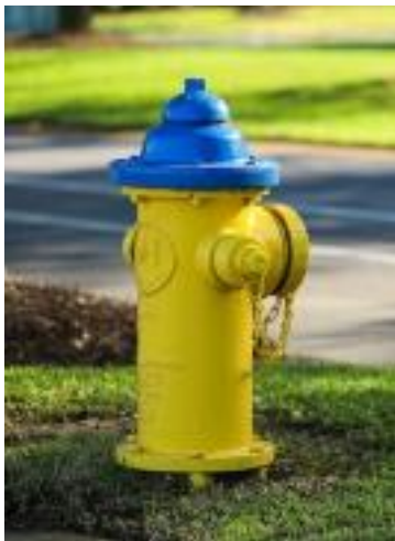
Figure 41: Properly colour-coded hydrant.
