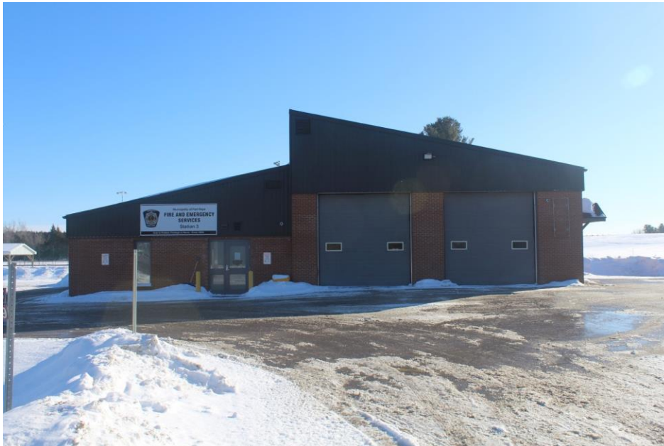
Figure 28: Fire Station 3 (Garden Hill).
