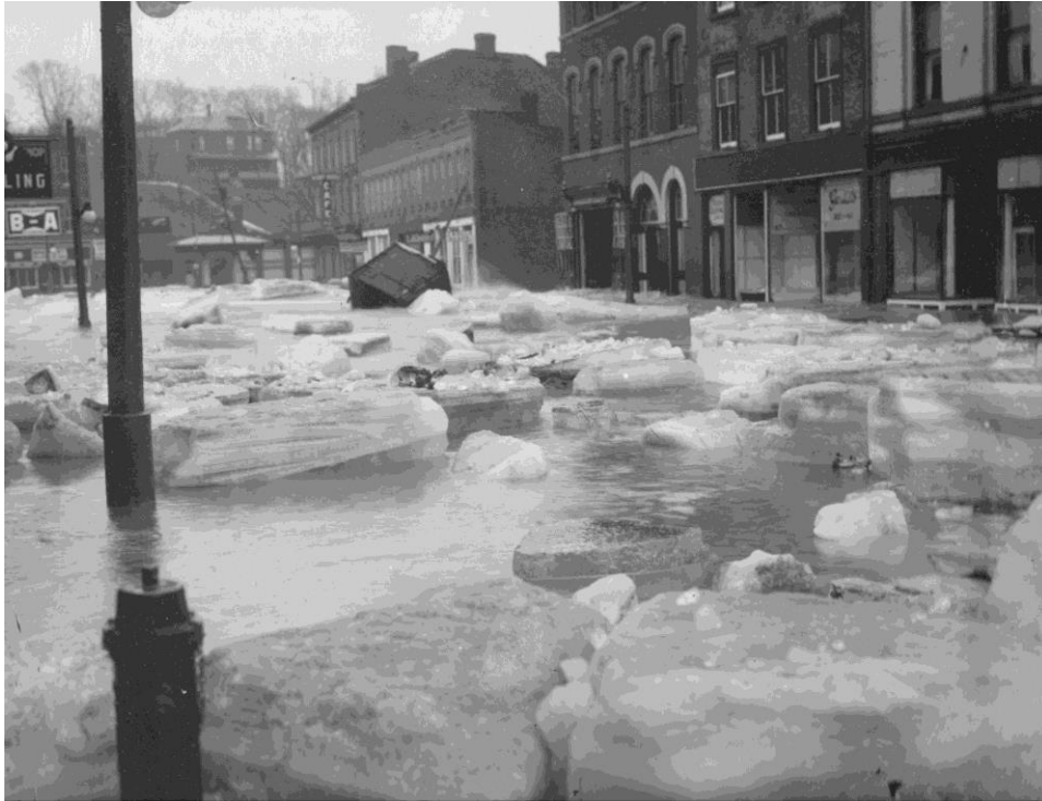
Figure 5: Flooding in downtown Port Hope.
