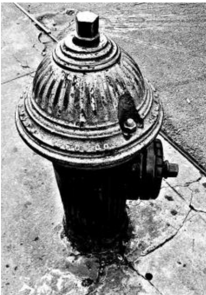
Figure 3: Fire hydrant in the downtown area.
