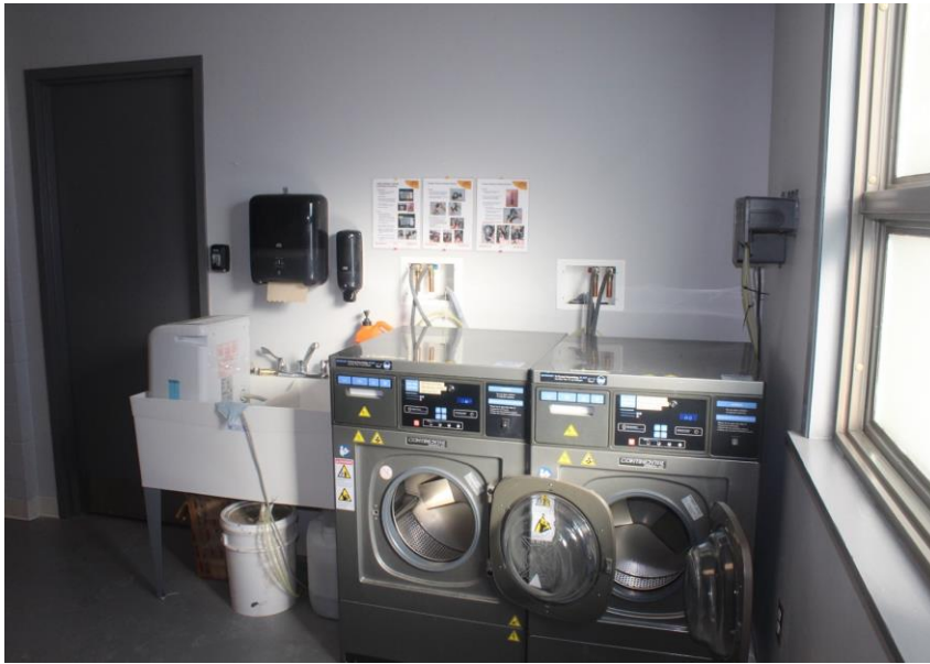
Figure 32: Bunker gear cleaning area at Fire Station 3.
