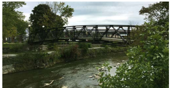
Existing Bridge Maintenance
