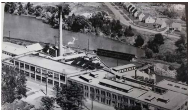
File Factory and former railway bridge over the Ganaraska, circa 1920
