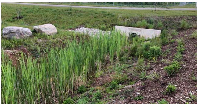
Natural Drainage System
