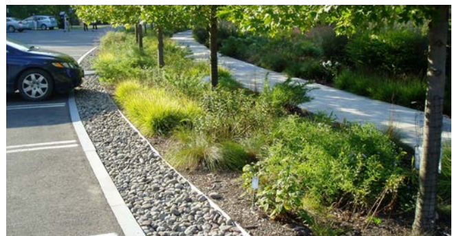
LID (Bioswales) incorporated into parking
