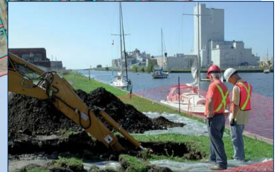
LLRWMO harbour wall soil investigations
