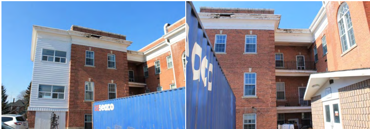
Figures 34 & 35: (left) View of east elevation of west wing, looking west (right)View of east elevation of west wing, looking west towards balconys/alcove (Source: MHBC, 2018)
