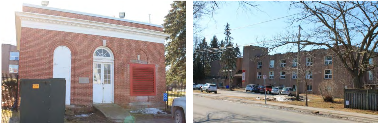
Figures 4 & 5: (left) View of ‘powerhouse’ / laundry facility looking south, (right) View of Hope Street Terrace looking south-west from Hope Street (Source: MHBC, 2018)
