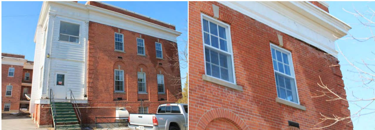
Figures 32 & 33: (left) View of east elevation, looking west (right) Detail view of stringcourse and windows at second storey of east elevation, (Source: MHBC, 2018)
