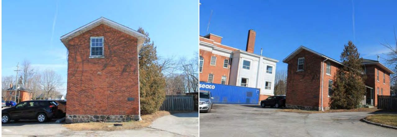
Figures 49 & 50: (left) View of west elevation, looking east towards second brick addition (right) View of south and west elevations, looking north-east (Source: MHBC, 2018)
