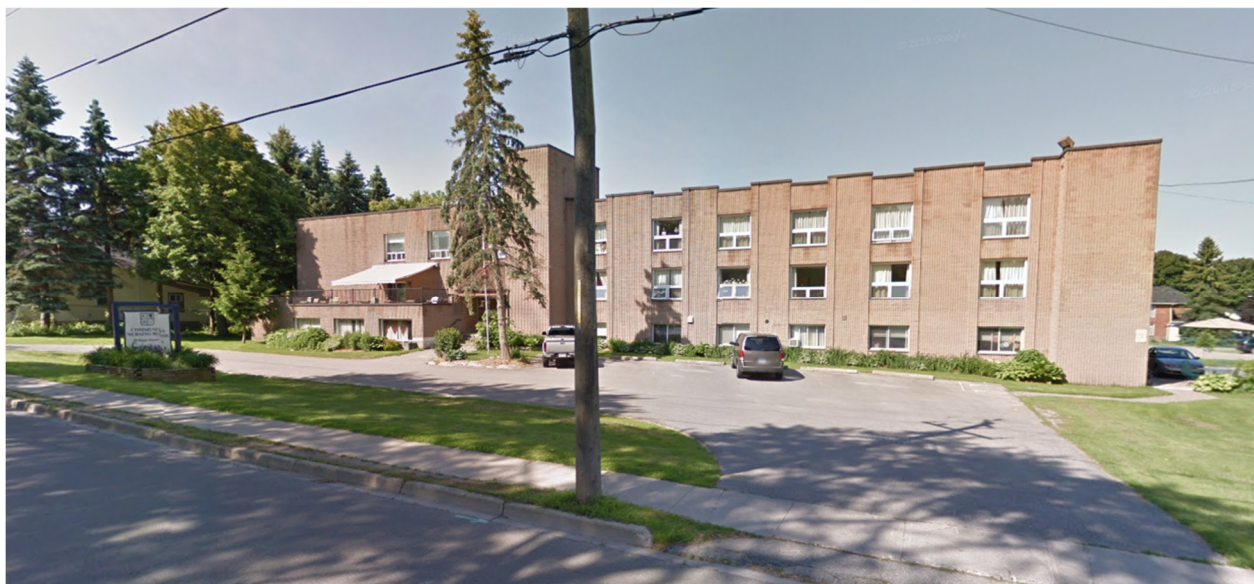
Figure 2: View of the Hope Street Terrace Long-Term Care Home from Hope Street
