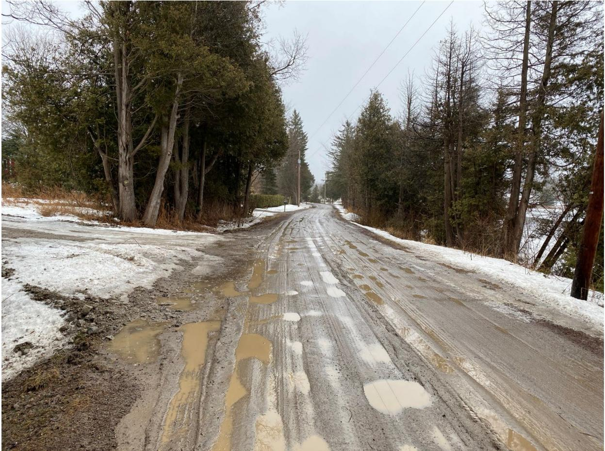
Monument conducted a topographic survey of Mill Street in September 2022. The extent of the survey was carried from the Ganaraska Road intersection for a total length of 1050m north past the extent of the Mistral property. The survey revealed a gravel driving platform of roughly 5.5m with very shallow ditching (~0.3m) along the east side of the roadway. The existing alignment is illustrated in the attached drawings (06).
