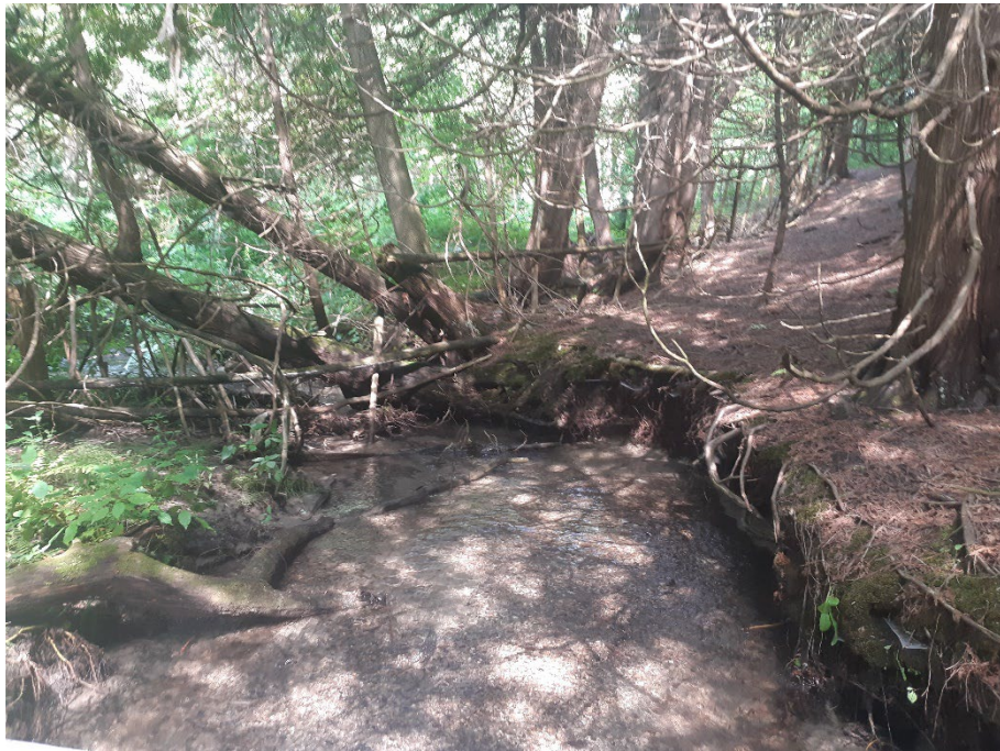
Photo 8 View of erosion scars of north watercourse within forested area, July 2021.
