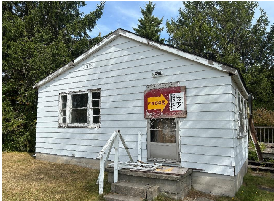
Photo 3 West portion of Site Building B, September 28, 2023.
