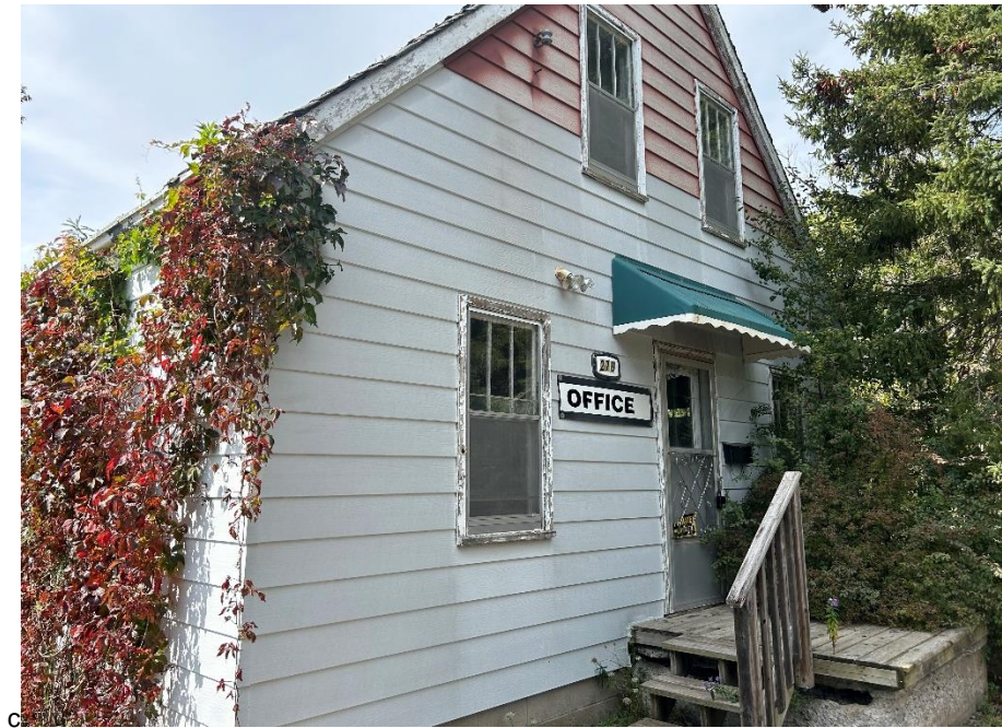
Photo 1 East portion of Site Building A, September 28, 2023.
