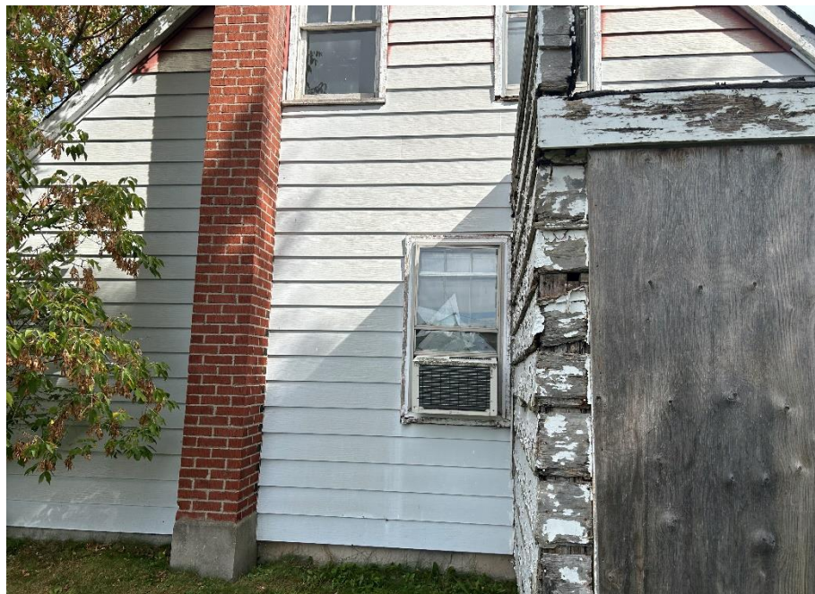
Photo 2 West portion of Site Building A, September 28, 2023.
