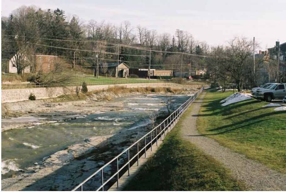
Above: View southeast along Ganaraska River, seen from Ontario Street.
