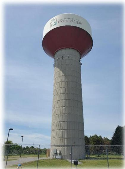
The **Fox Road elevated Tower** provides off-site storage tank that can hold up to 3,000 m<sup>3</sup> of water.
